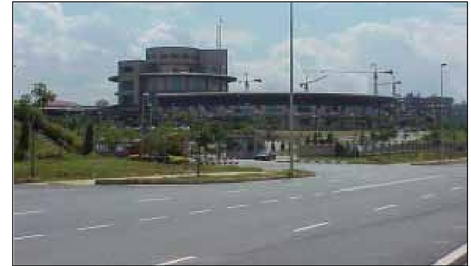
Photo 1.1: Road Leading To Precinct 7
