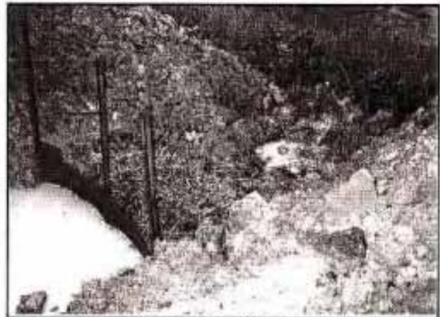
Figure 10.5 Use of Geofabric and hay bales
