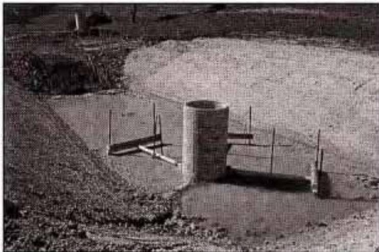
Figure 10.10 Floating skimmer system used in a sedimentation basin. The skimming system consists of three PVC T-pipes mounted on floats.
