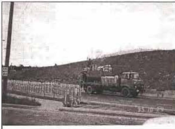
**Figure 10.2** Spraying of paper machee on embankment
