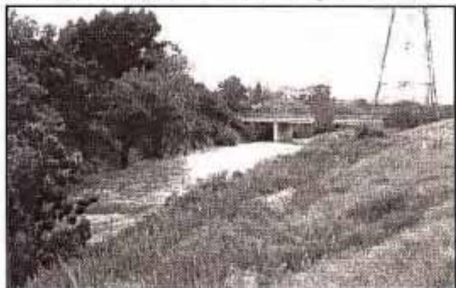
Figure 10.7 Buffer strip between exposed area and receiving waters
