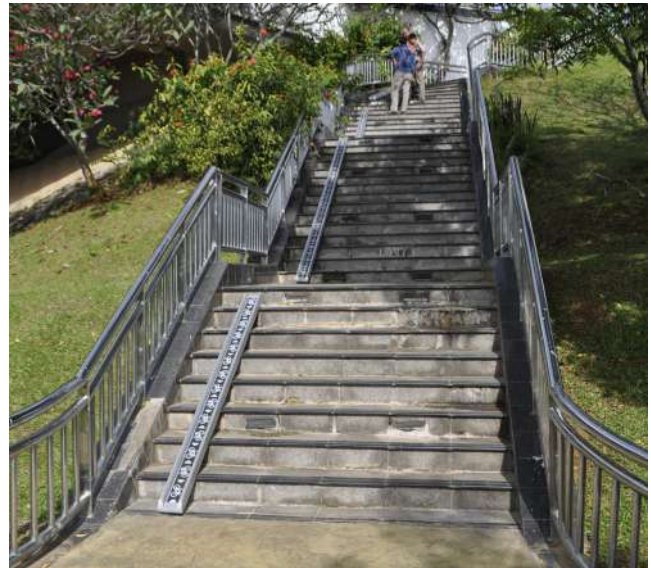
Bike access ramps installed at the staircase of Seri Wawasan Bridge and Seri Saujana Bridge.
