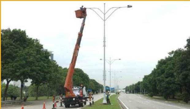
Installing LED street lights at Lebuh Wadi Ehsan
