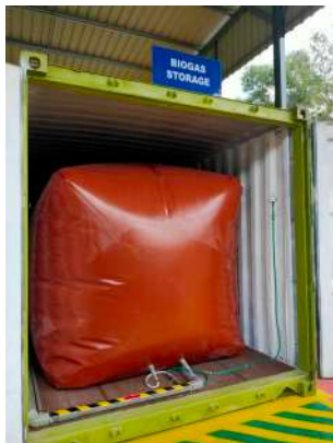
Biogas that had been produced is kept in this 20m 3 capacity storage bag.
