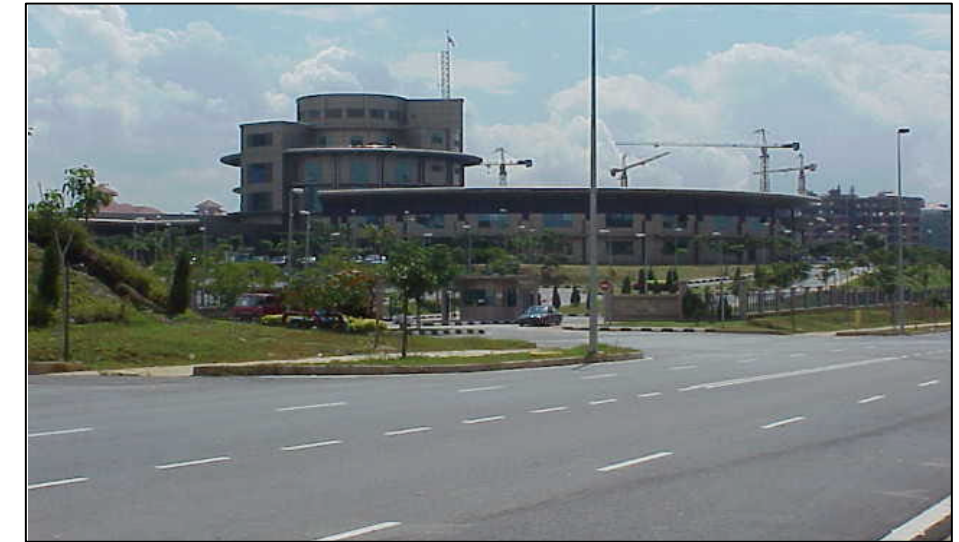
Photo 1.1: Road Leading To Precinct 7
