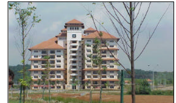
Photo 4.2 : Apartment in Precinct 9 is high density residential
