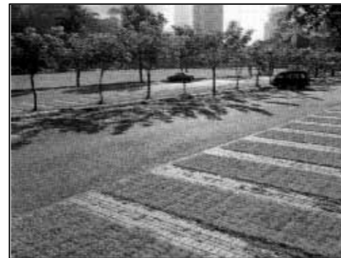
Figure 4.16 Pervious Surface for Parking Area
