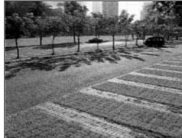
Figure 3.34 Use of Pervious Pavement at Parking Area
