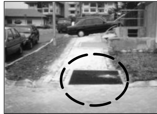
Figure 4.18 Grille Shall Be Properly Positioned to Avoid Difficulty For Walking
