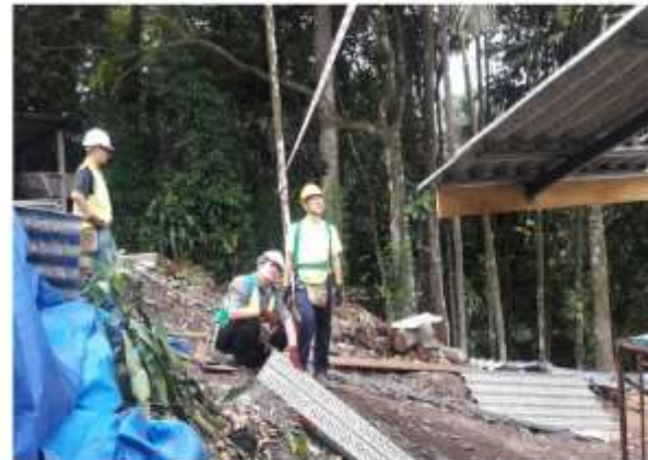
Builders checking alignment of the roofing installation
