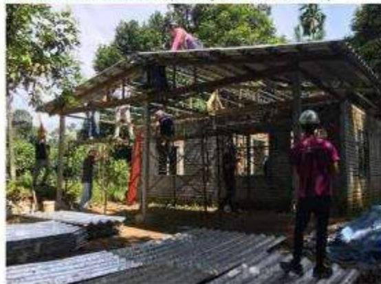
Abang Faizul Roof Construction - Kg. Sg. Lalang, Semenyih In collaboration with Buildables (formerly known as Platform 80)
