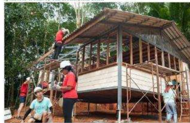
EH 106 - 6 Modules Asli Home for Pak Din & Wah Risan family sponsored & built by Gen T. Malaysian Tatler
