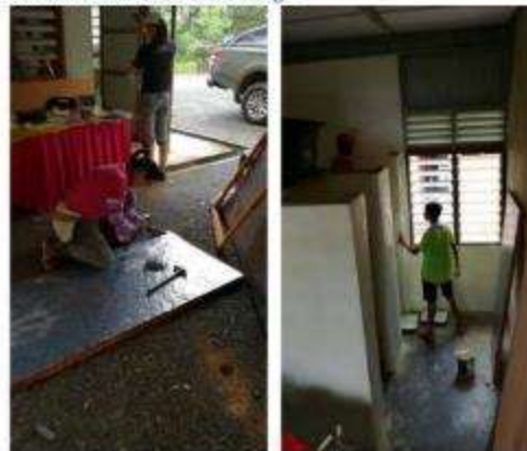
Refurbish Community Centre at Tangkak, Johor In collaboration with Small Changes
