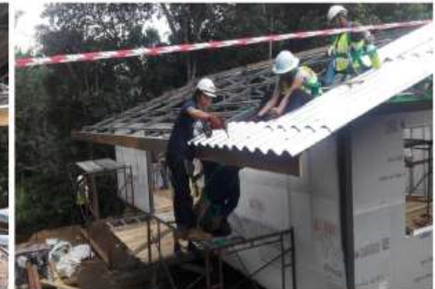
Builders installing the roof sheets onto the purlins
