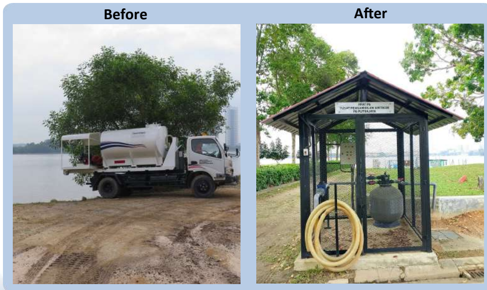
Lake water intake station, Precinct 6
