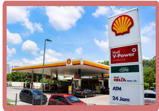
Shell Petrol Station, Precinct 18 (GBI – Certified)
