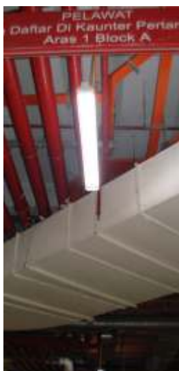
T6 fluorescent light fixtures are widely used in the basement parking area
